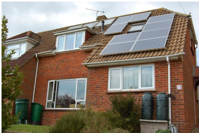
Solar Thermal & Solar PV Panels
