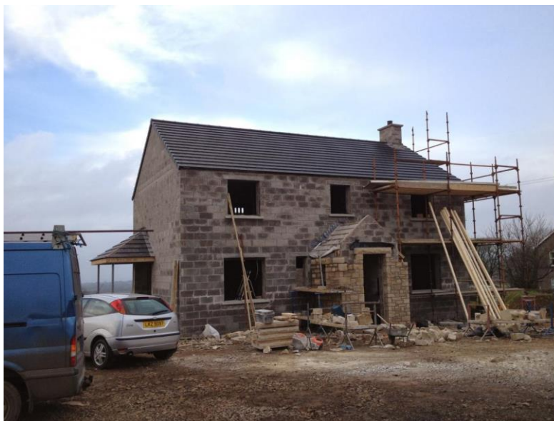
FmK ECOHome No.02 - under construction
