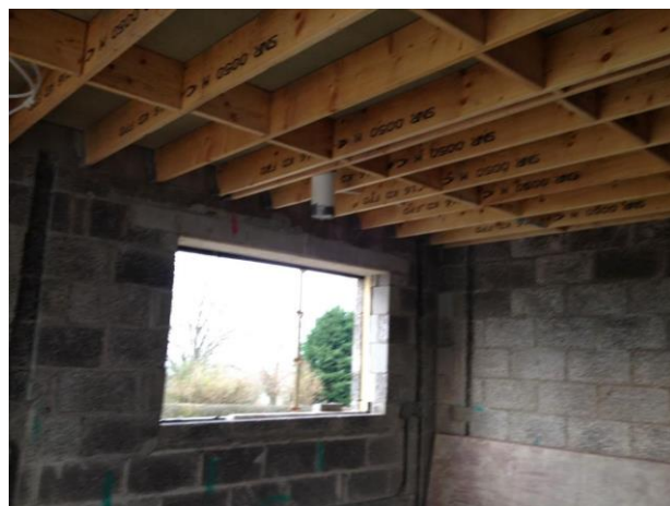
Timber Floor Joists
